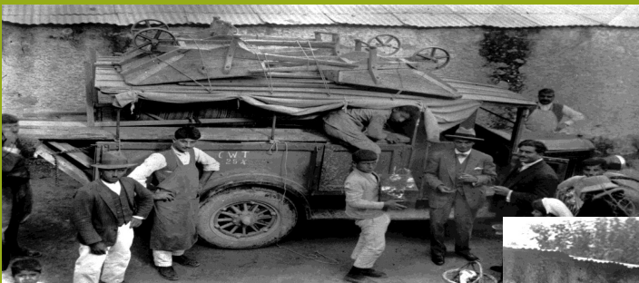
Note the wooden wheelbarrows on top of the lorry. Sjöqvist, smoking a cigarette, supervising the work
