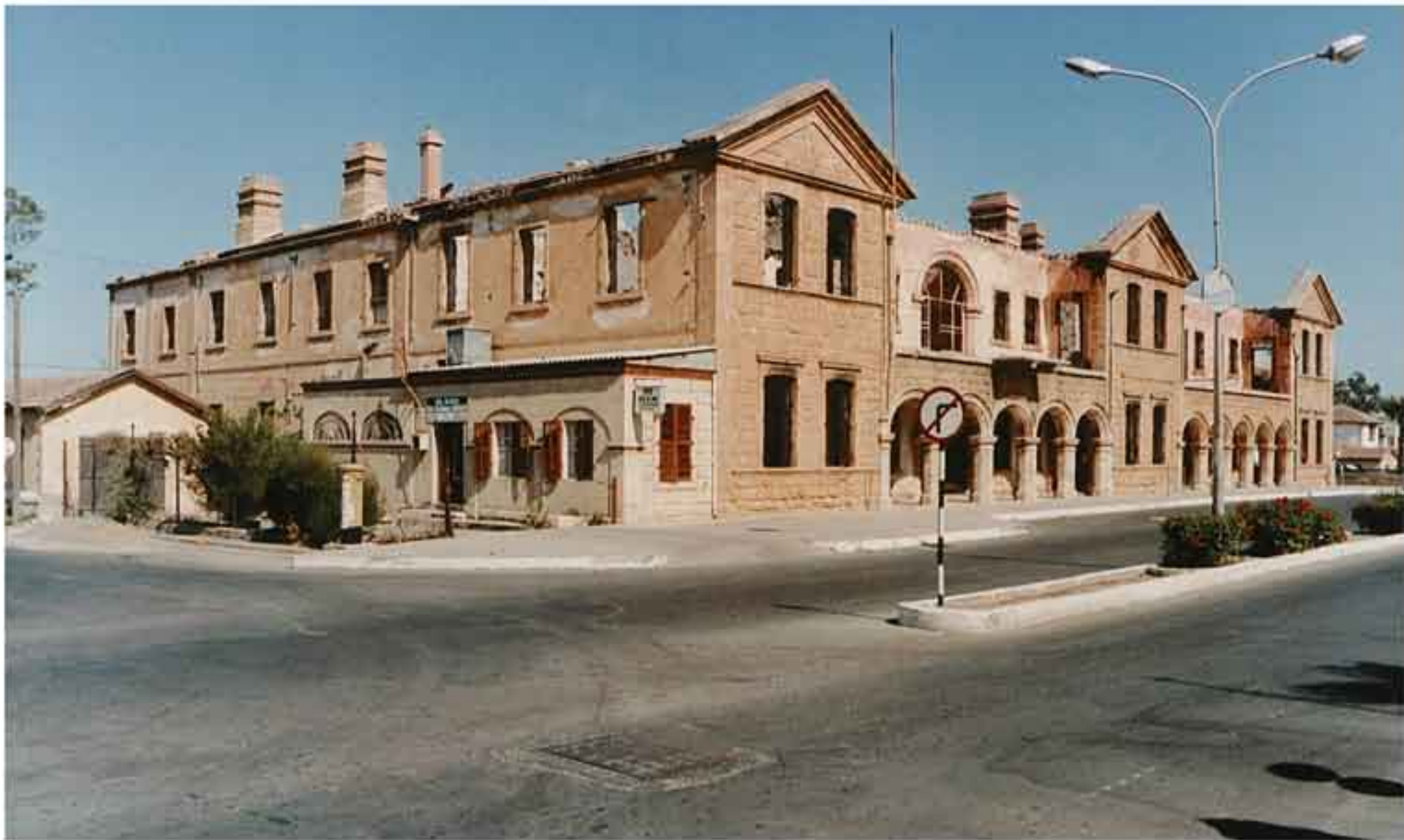
The District Office of Famagusta after being bombed in 1974.
